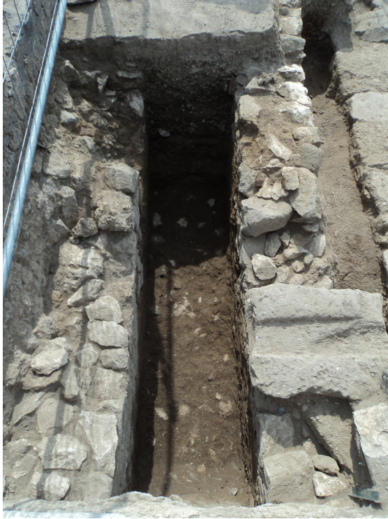
Fig. 3 - Sewer canal along the eastern stylobate, from the north.
